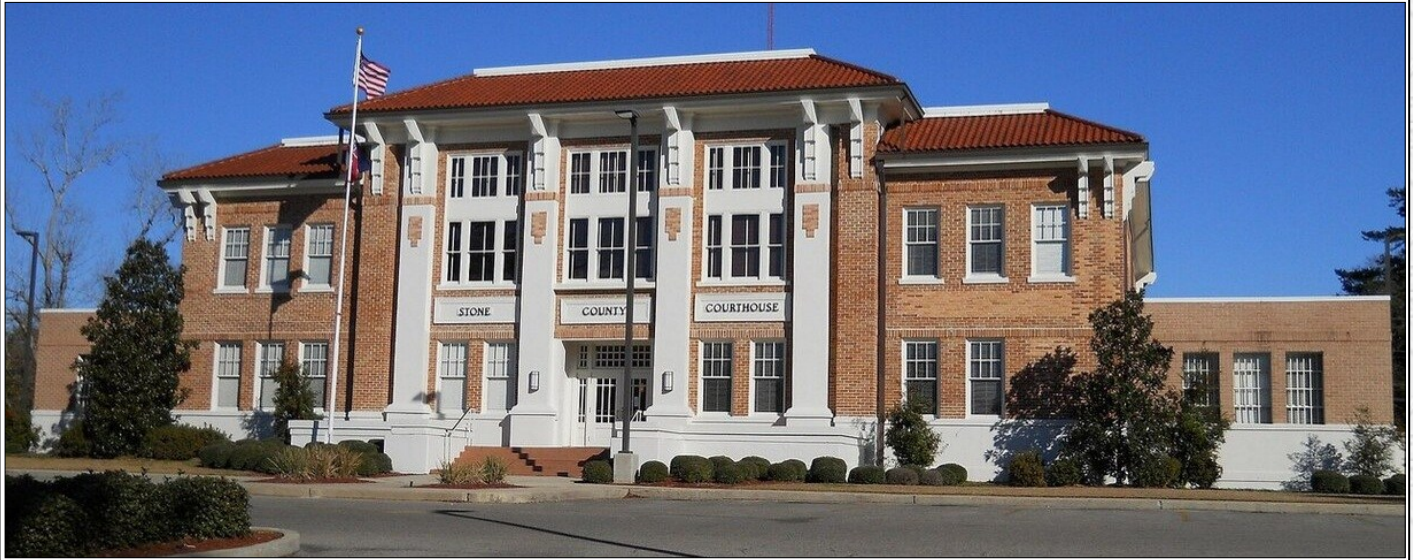
Stone County Courthouse in Wiggins, Mississippi. Stone County was named after John Marshall Stone. | public domain
