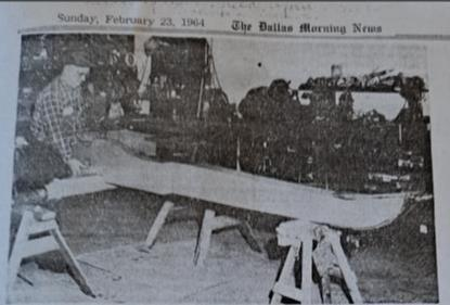
"Old Valverde"—a Union cannon which "Texas Confederates turned into a Yankee-killer—comes back to life in the shop of Phil Wetherhold at Teague. The 7-foot-long redwood "trail" Wetherhold is assembling in picture is the largest part of a brandnew gun carriage he is constructing.
